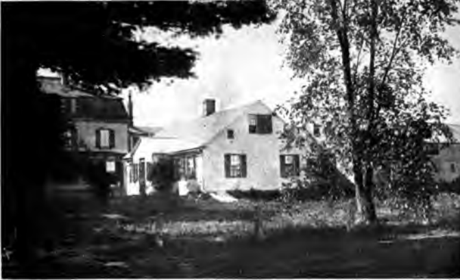
HOUSE IN WHICH WEBSTER LIVED AT DARTMOUTH, NORTH MAIN STREET
